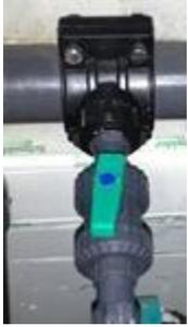
At the end of the hose discharge line carrying the chemical from the dosing pump, the water should be added with a clamp from a point where it will not come into contact with any equipment after that point. **If water containing dense chemicals comes in contact with any equipment, it may cause irreversibly damages.**
