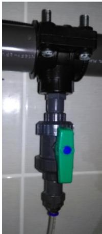
After measure water, measured water is injected to return line with a clamp settle.
