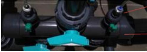
The sample is taken from the water and sent to the flow cell for measurement and returned to the system.
