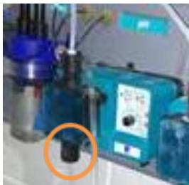
The hose from chemical tank is connected to the lower hose connection of the dosing pump.
