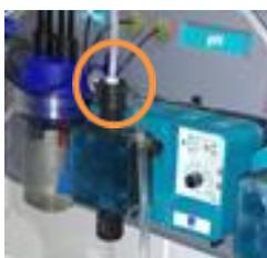
The upper hose connection of the dosing pump is the connection to the pool. After this, the chemical is given to the pool water.
